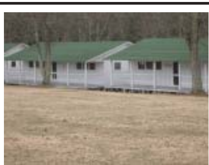
The new porch railings on the bunks of Mason and Morgan.
